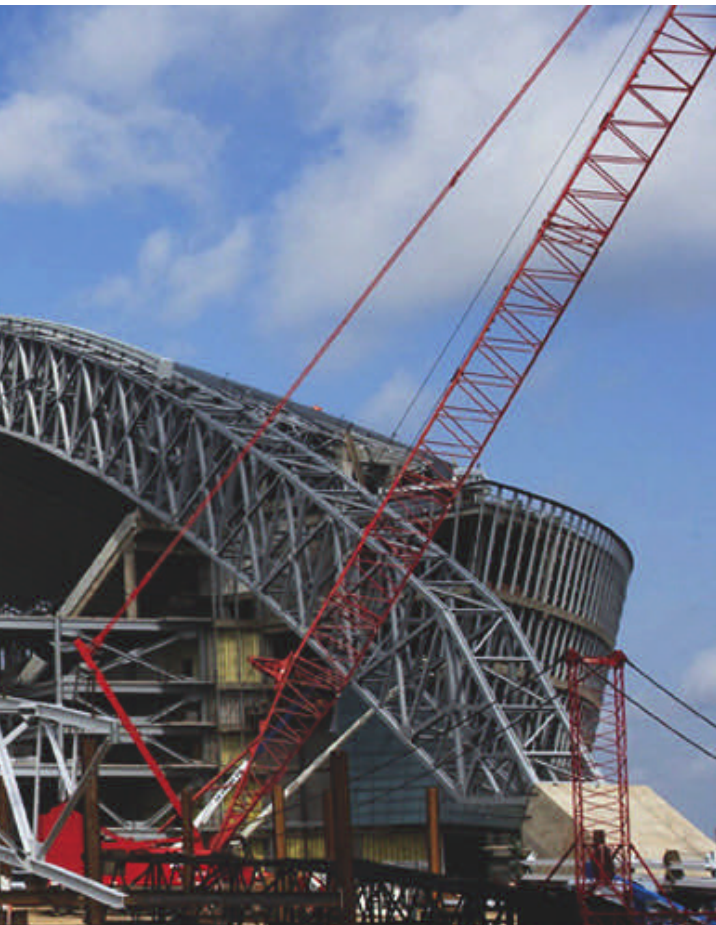
A crane hoists a segment of one of the six box trusses into position between the soaring twin arch trusses.
