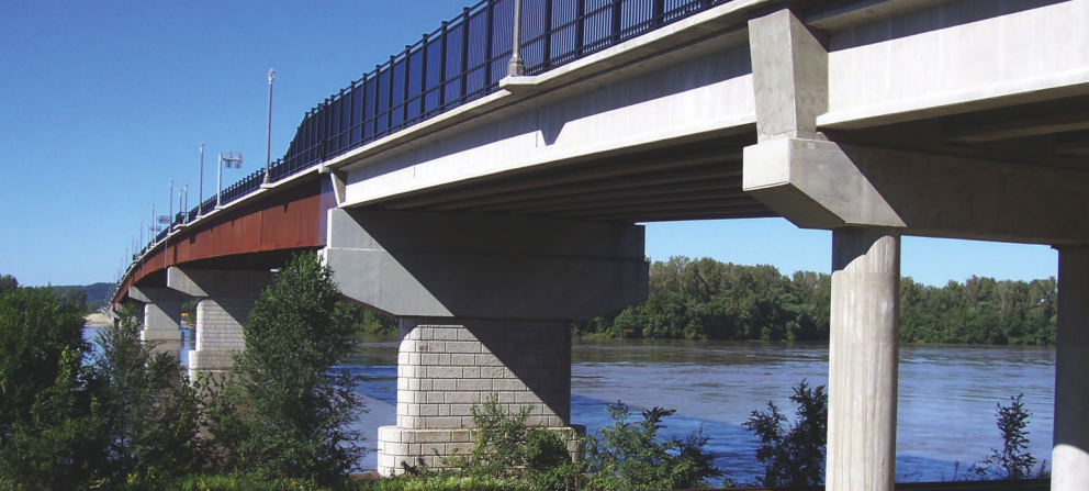
High-performance steel was used for the negative moment flange plates over the piers.
