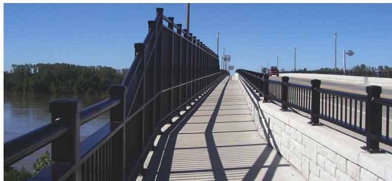
Ornamental pedestrian fence and handrails made from hollow structural sections adorn the new Christopher S. Bond Bridge.
