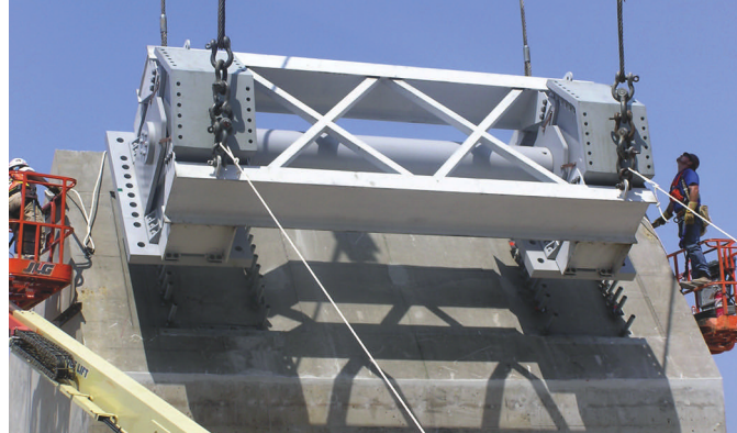
A 64,000-lb cast steel pin assembly touches down on one of four massive concrete abutments that transfer 19 million lb of thrust from an arch truss into the ground.
