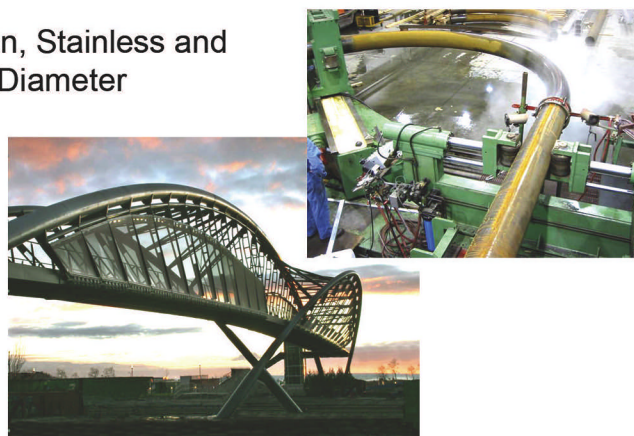
"Helix Bridge" Seattle, Washington 36" OD x 1.25" wall & 24" OD x 1" wall cold bent to a multiple radius helix
