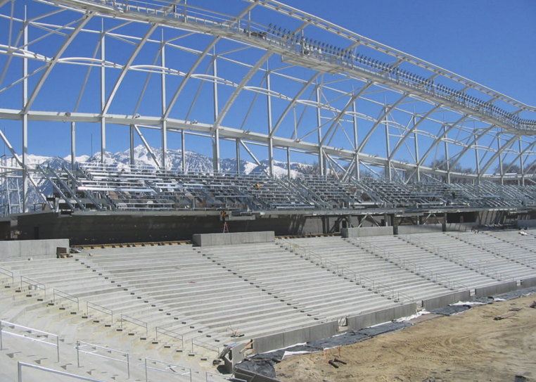
Roof framing before canopy installation.
