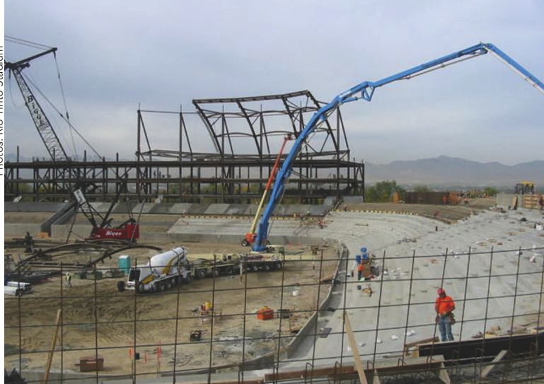
Erection of the canopy framing.
