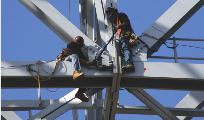
Ironworkers tighten bolts in one of the slip-critical end plate splice connections that link the 56-ft long segments of the arch truss chords.
